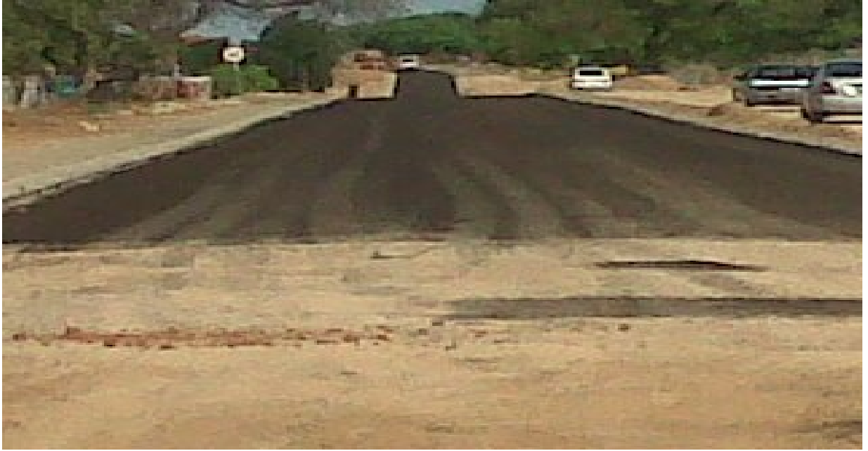
Picture 2: Road construction at Mkhuhlu Main Street leading to Calcutta village.
