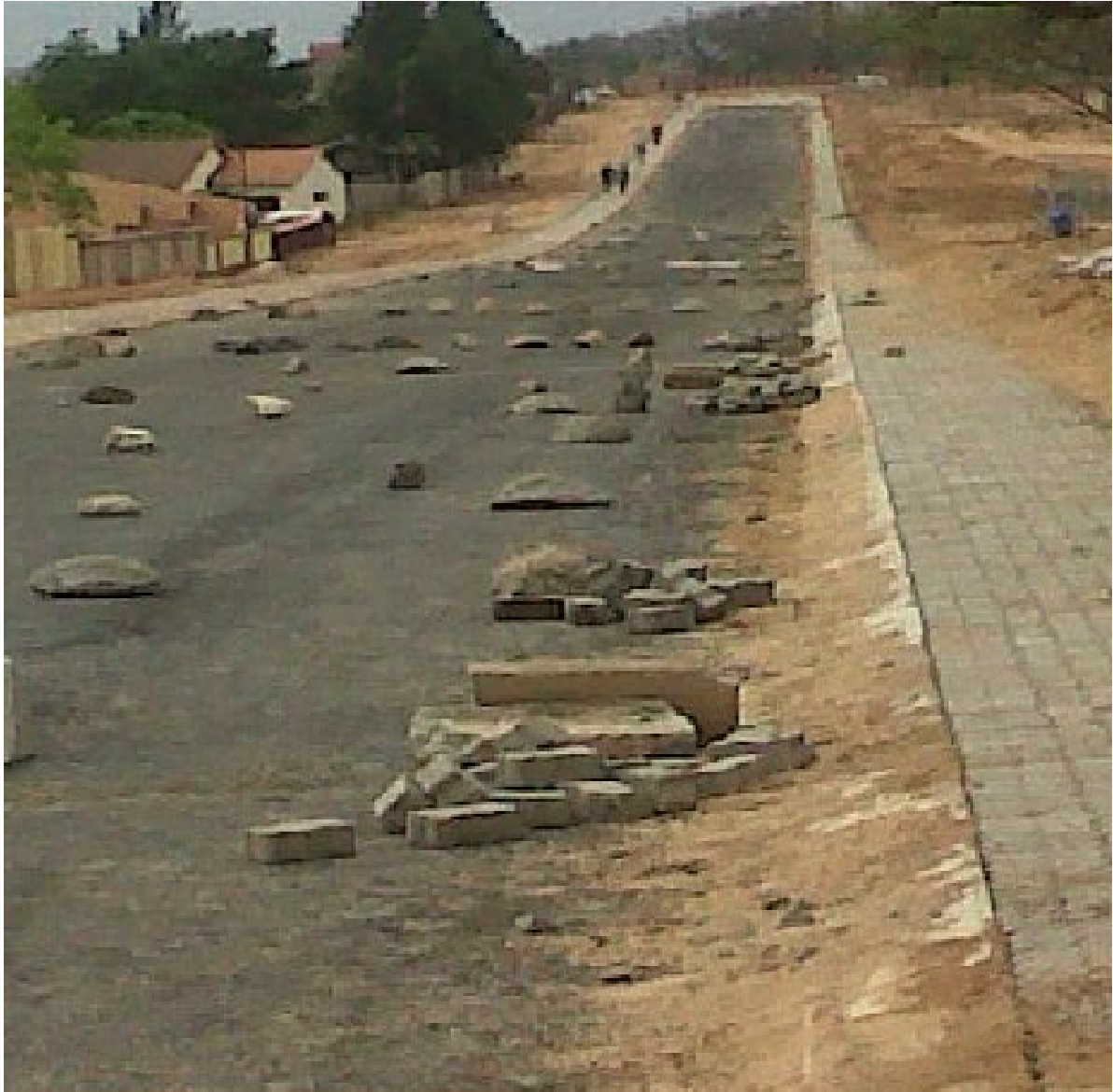
Picture 4: Road construction at Mkhuhlu Main Street towards Calcutta village.
