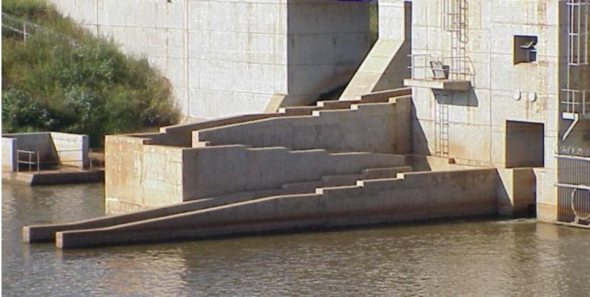
Figure 8. 6: The construction of the Xikundu fishway in the Luvuvhu River.
