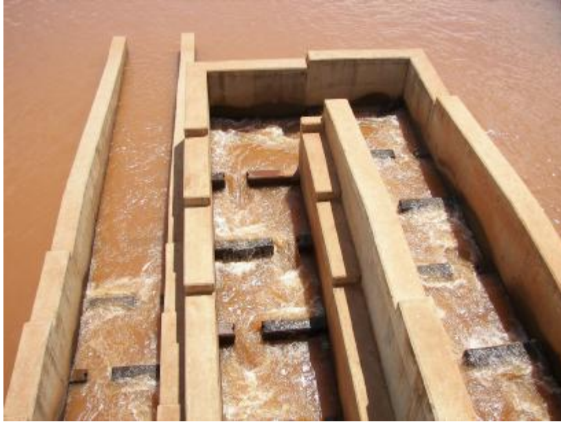
Figure 8.21: An illustration of the volume of water in the Xikundu fishway during the February 2006 survey.
