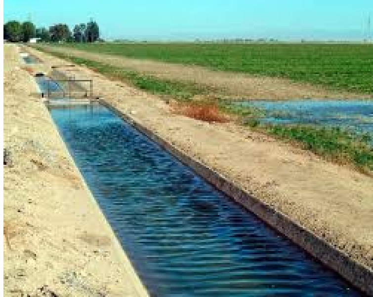
Figure 1.3: Example of open channel flow(Image source: civiltoday.com)
