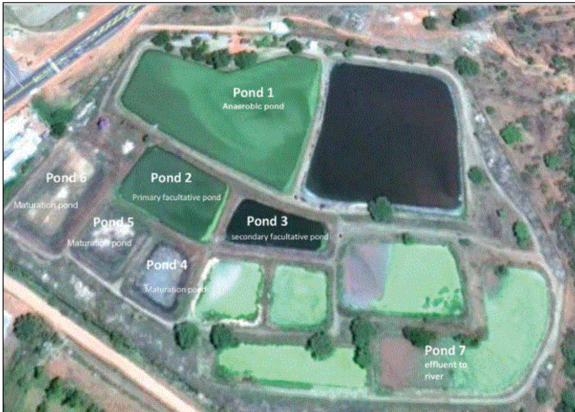
Figure 2.2: Layout of the ponds at Motetema wastewater treatment plant (from Genthe & Oberholster 2016).
