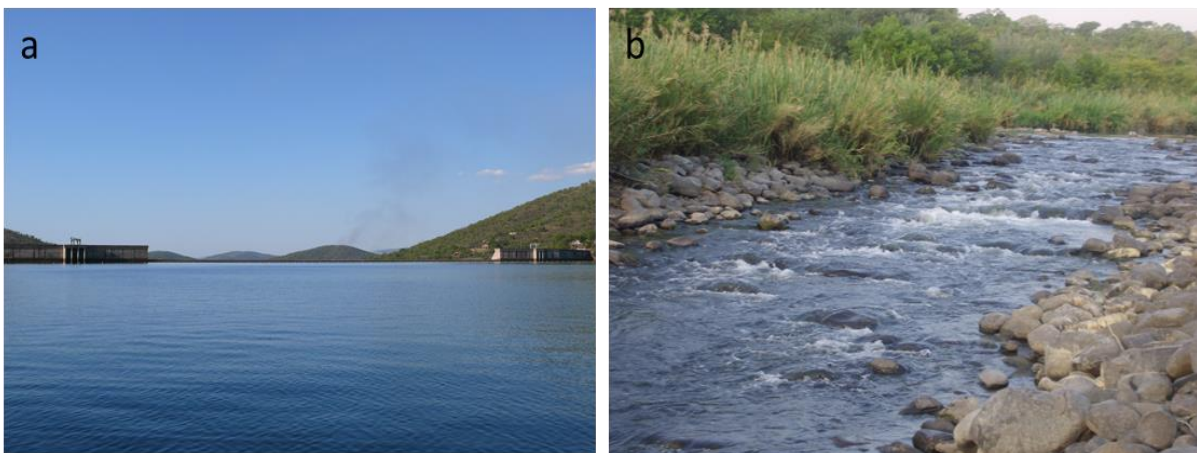
Figure 2.5 a. Loskop Dam wall; b. Loskop Dam inflow with reeds on the edge.
